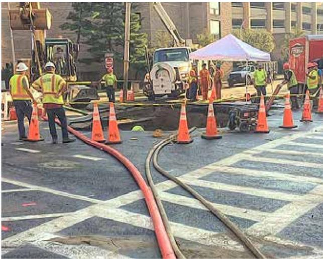
The crater on the left, just down the block from the White Plains Library, resulted in disruption last month to drivers, pedestrians and water users when a ruptured water main caused a major street to collapse.
